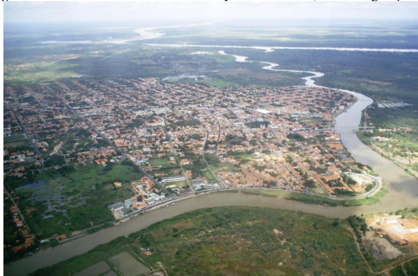
Figure 7 - Construction of homes in the city of Parnaíba-PI, near the Igarçu river
