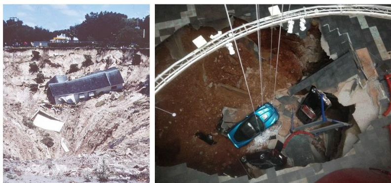
Figure 11 - Left) Winter Park Doline, Florida: source: Anthony Navoy, USGS. Public domain; Right) Doline collapse under Corvette Museum, Kentucky, USA
